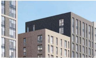
During the latter stages of development parts of each façade were amended and simplified for ease of construction. The composite stone frame has been replaced with a similar coloured brick to maintain the distinctive grid pattern whilst reducing the weight and cost of the previous system. The brick system used includes a glazed brick infill from the 19th storey upwards to maintain the hierarchy of the façade and definition of a 'crown'.
